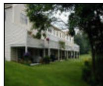
The decks at this New Hampshire condo property are a good example of why the 1980s earned a reputation for poor quality construction. The use of untreated lumber contributed to the rapid deterioration of the decks. John Turner, P.E., of Criterium-Turner Engineers was assigned the mission to identify "What went wrong?"
